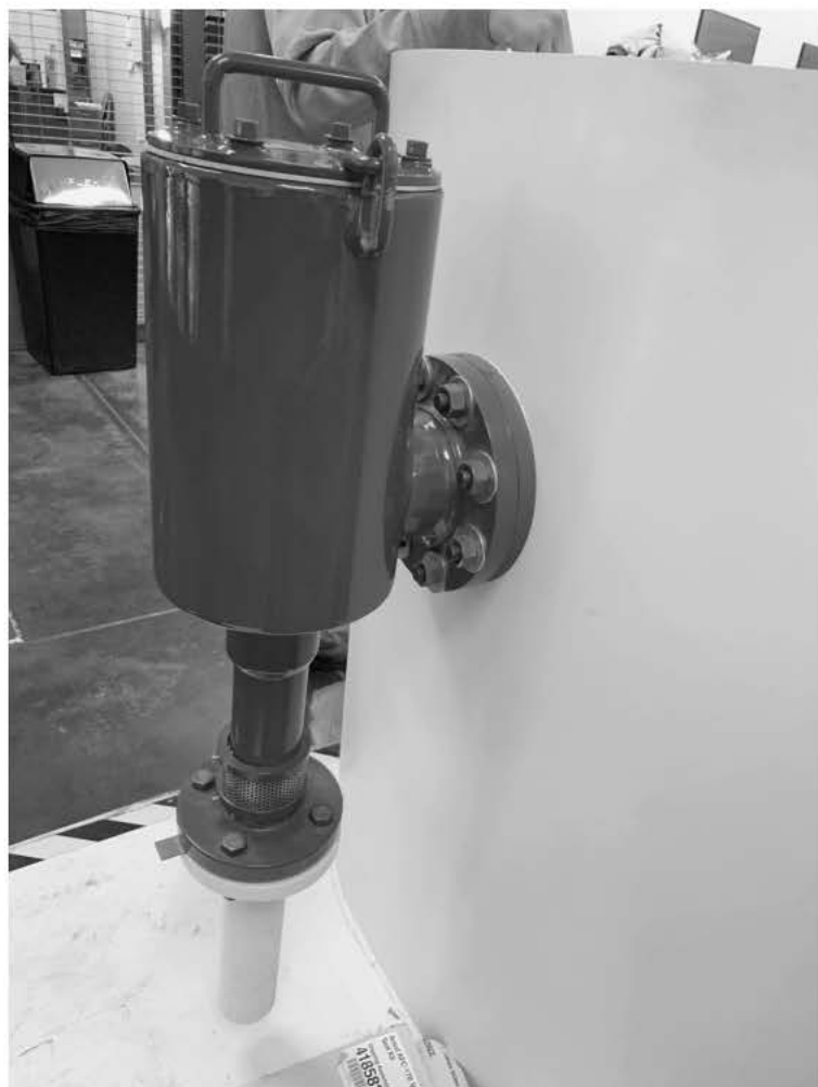
FIGURE A.5.2.5.2.1(a) Foam Chamber.
