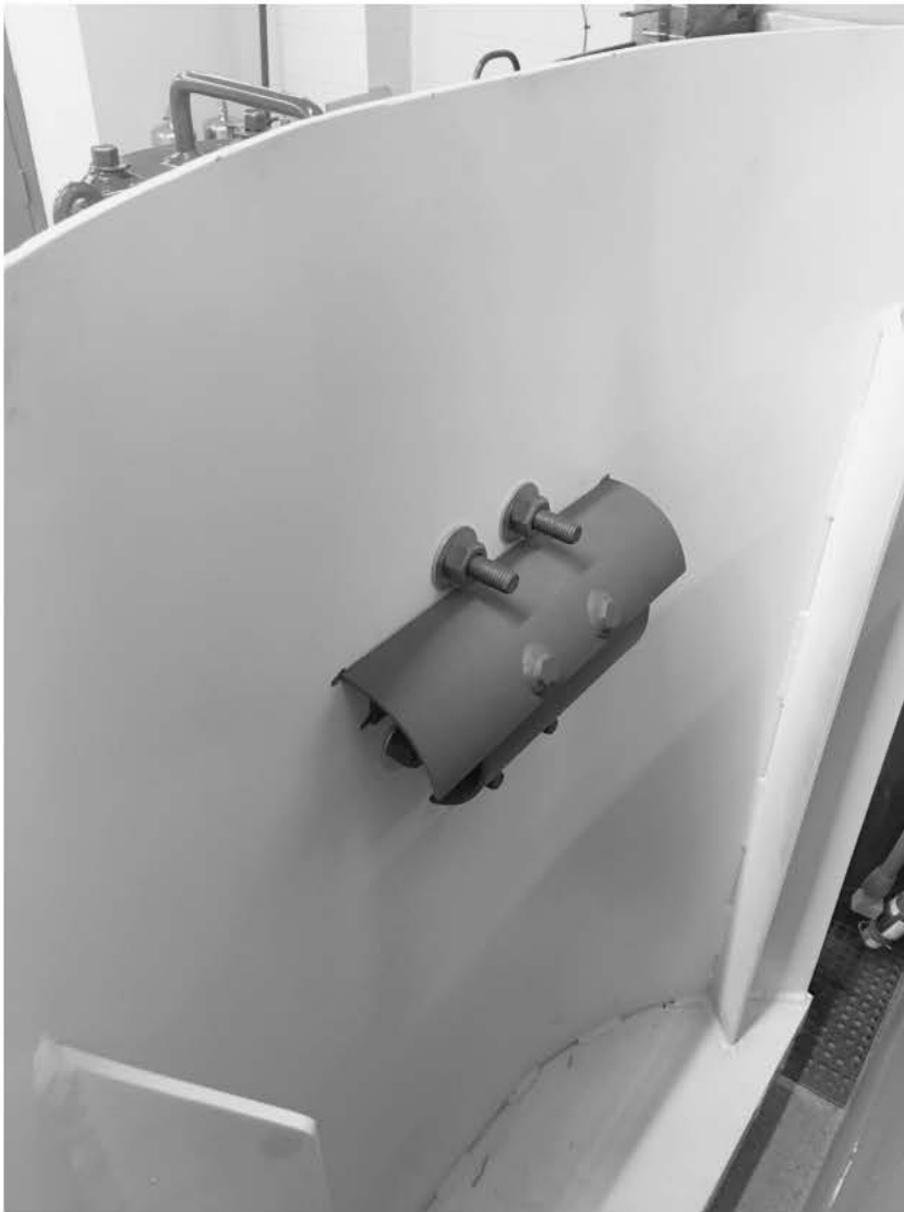
FIGURE A.5.2.5.2.1(b) Foam Chamber Deflector.
